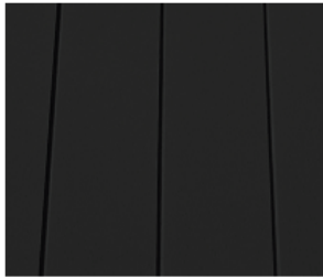
Dark coloured vertical cladding to the upper levels of both houses
